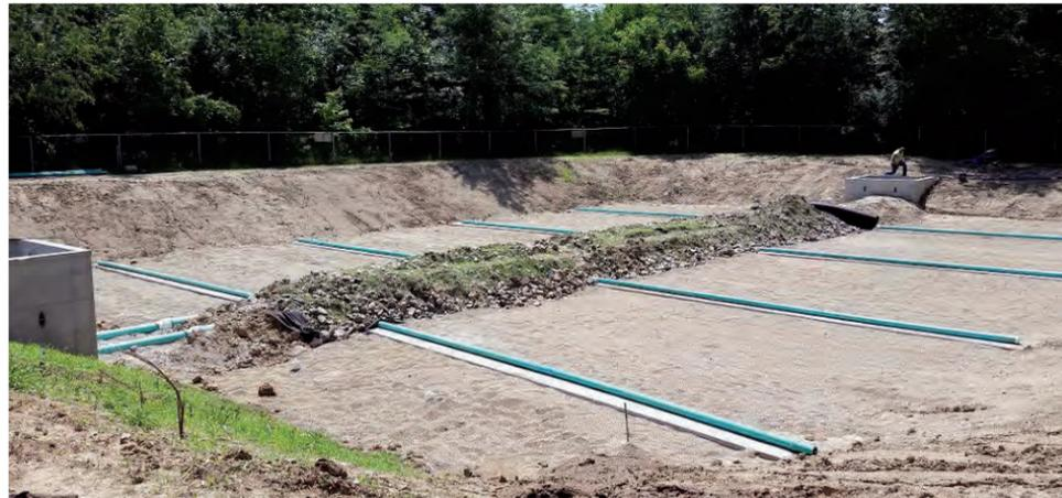
Work is continuing at the Funks Grove rest area and is on schedule as of this printing. The contractors have completed pumping and repairs to the septic holding tanks near the main building and are currently working on the new sand filters. The sand filters are the last stage of the lagoon system. Soon they will begin work on lagoons one and two. Pictured is the new sand filters in progress.
