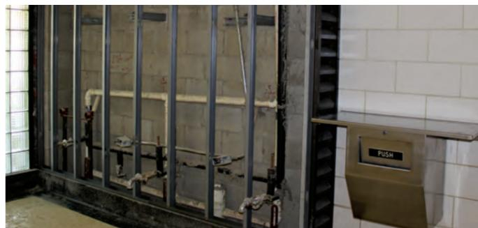
Sink wall after the glazed tile block wall has been removed. Notice the new framing already installed in preparation for the plumbing work. This wall will be finished in a square ceramic tile similar in color to the existing glazed tile block wall.
